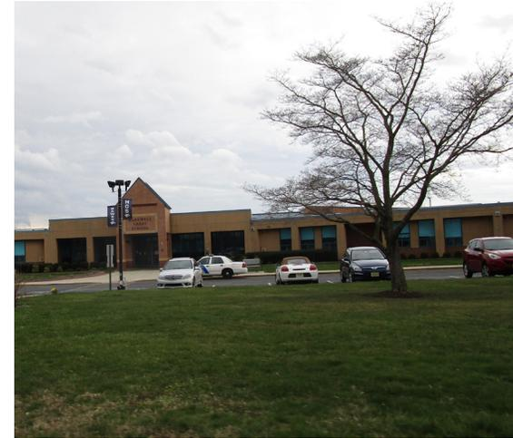
A rain garden can be installed on the west side of the parking lot on the west side of the property to capture, treat, and infiltrate stormwater runoff from the parking lot. A section of parking spaces in the east parking lot can be replaced with pervious pavement to capture and infiltrate stormwater runoff from the parking lot. A preliminary soil assessment suggests that the soils have suitable drainage characteristics for green infrastructure.
